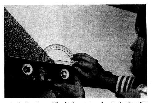
Fig. 7. Measuring roof angle, using level and protractor.
