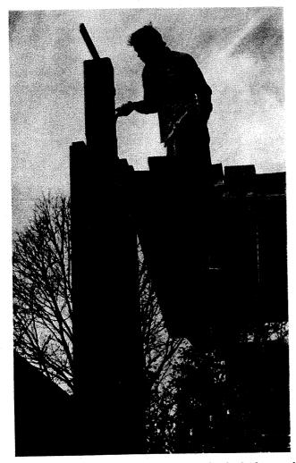
Fig. 12. Flue liner is placed first and the bricks laid around
