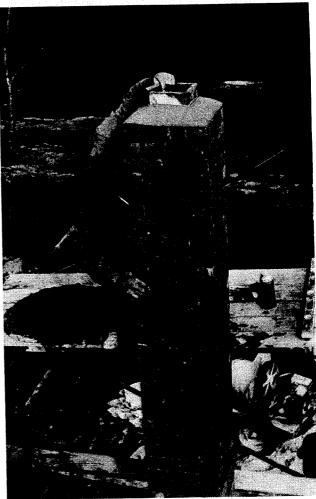
Fig. 21. Tooling the final mortar joints after topping out the chimney.
